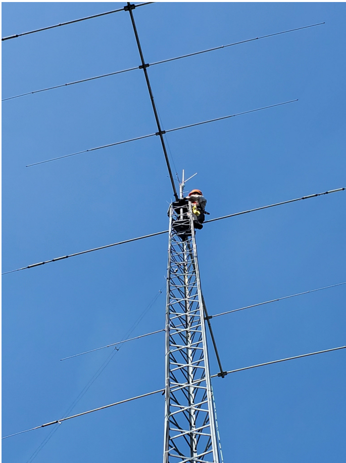
Devan VE7LSE making heading adjustments to VE7IADs TH6 beam.
