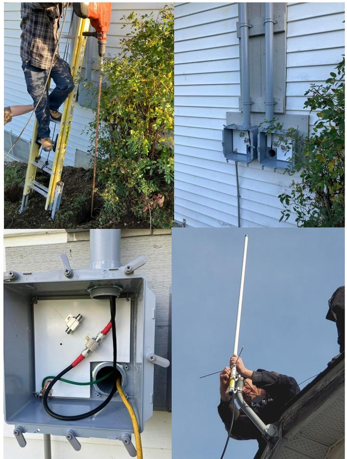
*Putting in the grounding rods at VE7NA and finalizing the antenna, rotator cables and CAT 5 entry boxes*
