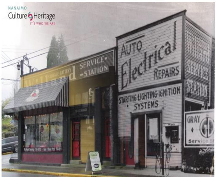
Sparks Co., the site of station CFDC, at 299 Wallace Street in downtown Nanaimo. The station transmitter would have been located in the upper level of the building at right. Willard was simply a popular US-made automobile battery brand, and the Sparks Co. sign is over the entrance door facing the corner of Fitzwilliam Street and Wallace Streets. (From the City of Nanaimo website)
