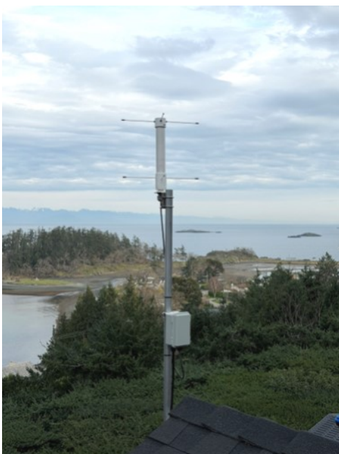
The view from the UHF turnstile antenna built by Bruce VE7PTN. It has excellent horizon to the east and north.
