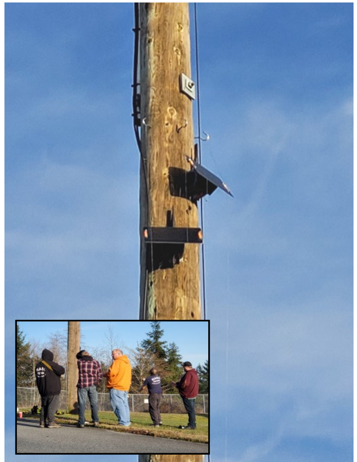
Kevin VE7KGV adjusting the final position of the solar powered Meshtastic and Meshcore nodes on the VE7NA hydro pole. Four NARA members provide encouragement!
