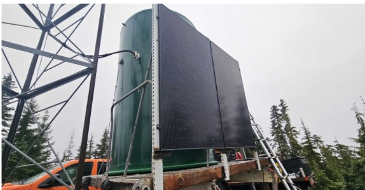
The two 450 watt solar panels at the new Woss ITS site.
