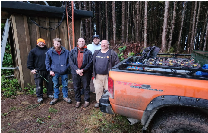
The battery installation team on Dec. 28. Left to right, Kevin, Jordan, Stuart, Mason and Randy.
