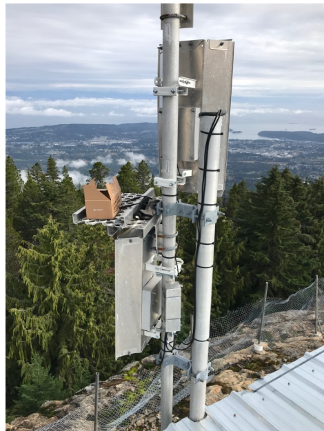
Two new Rocket transceiver units being fitted to the NARA 10 GHz AREDN node at Mount Benson.
